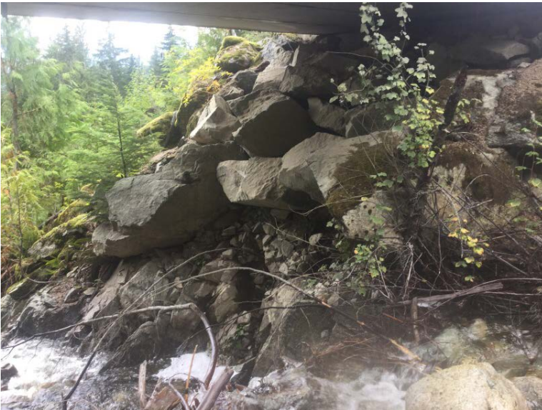
Right Bank Abutment when facing downstream
