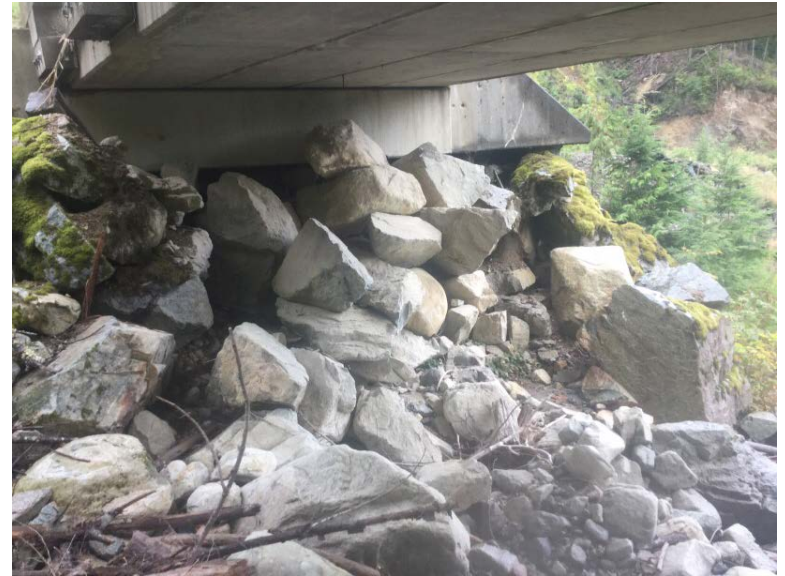
Left Bank Abutment when facing downstream
