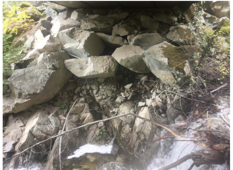
Right Bank Abutment when facing downstream
