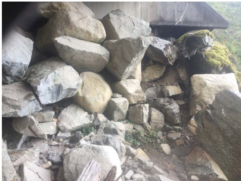
Left Bank Abutment when facing downstream
